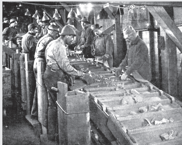
Figure 20: (Left) Workers sort ore by hand in the early years at Trail. (Right) A worker samples a flotation tank at Kimberly, c. 1960. (Cominco, 1960, 5, 10)
