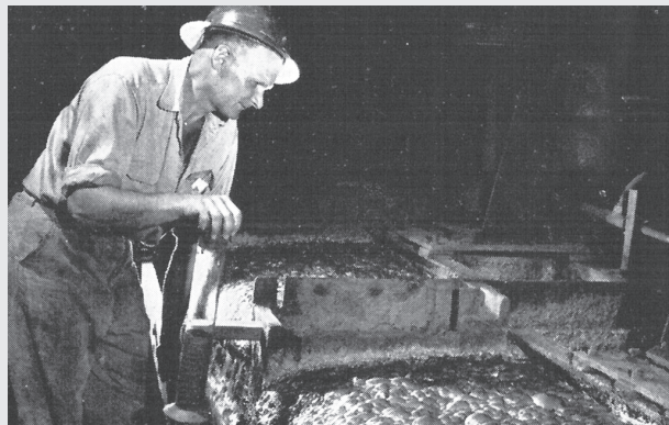
Figure 20: (Left) Workers sort ore by hand in the early years at Trail. (Right) A worker samples a flotation tank at Kimberly, c. 1960. (Cominco, 1960, 5, 10)
