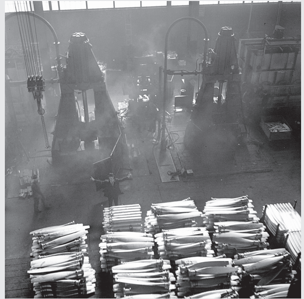
Figure 16: Propeller production at Alcan's Kingston plant in January of 1943 (Ronny Jaques/Library and Archives Canada/National Film Board Fonds, e000762922)
